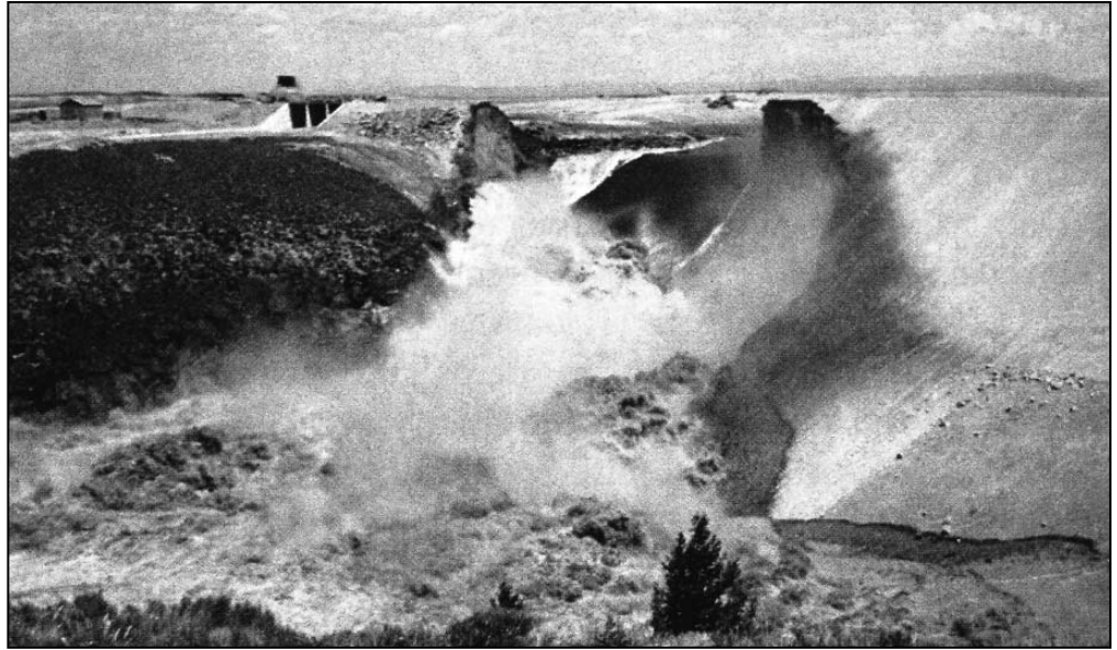
Figure 3. Failure of the Teton Falls Dam in Idaho, USA. The face of the loess dam is on the right, with the rock canyon wall on the left. The core of the dam has just totally collapsed into the piping cavity that had progressively enlarged along the original line of seepage through the permeable loess. (With thanks to the unknown photographer)
