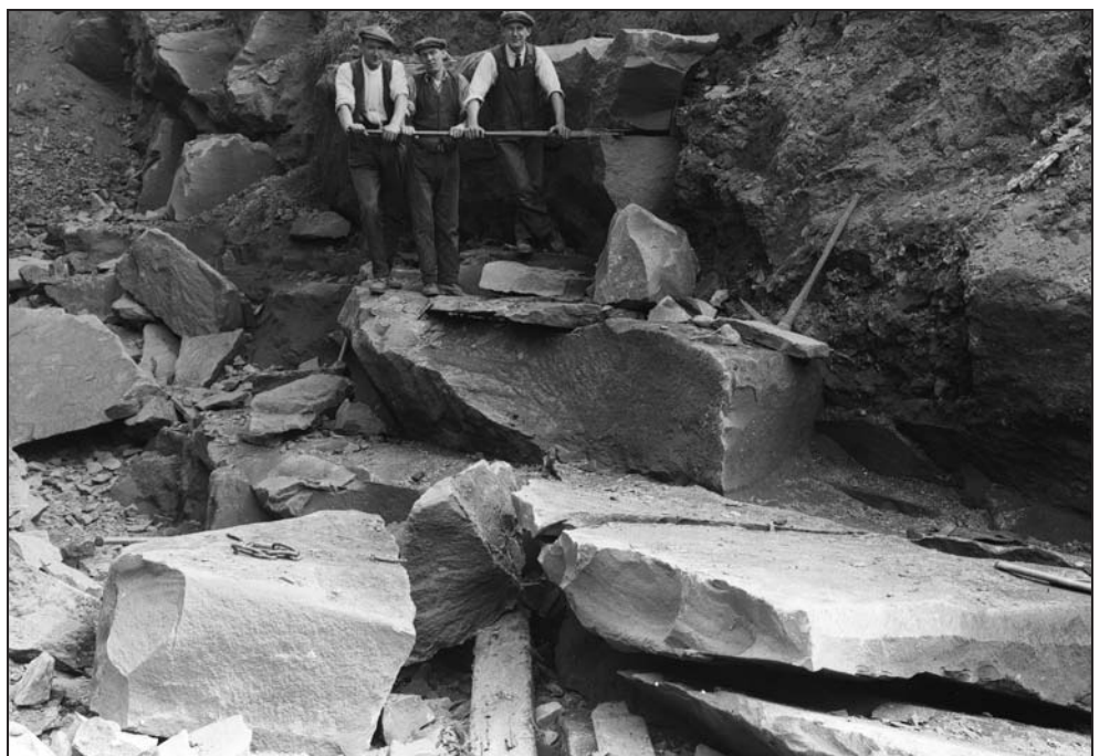
Figure 4. Lindley's Mansfield Red Quarry, at Mansfield: hand-working the dolomitic red sandstone of the Cadeby Formation. (BGS photo #A5053, 1930).
