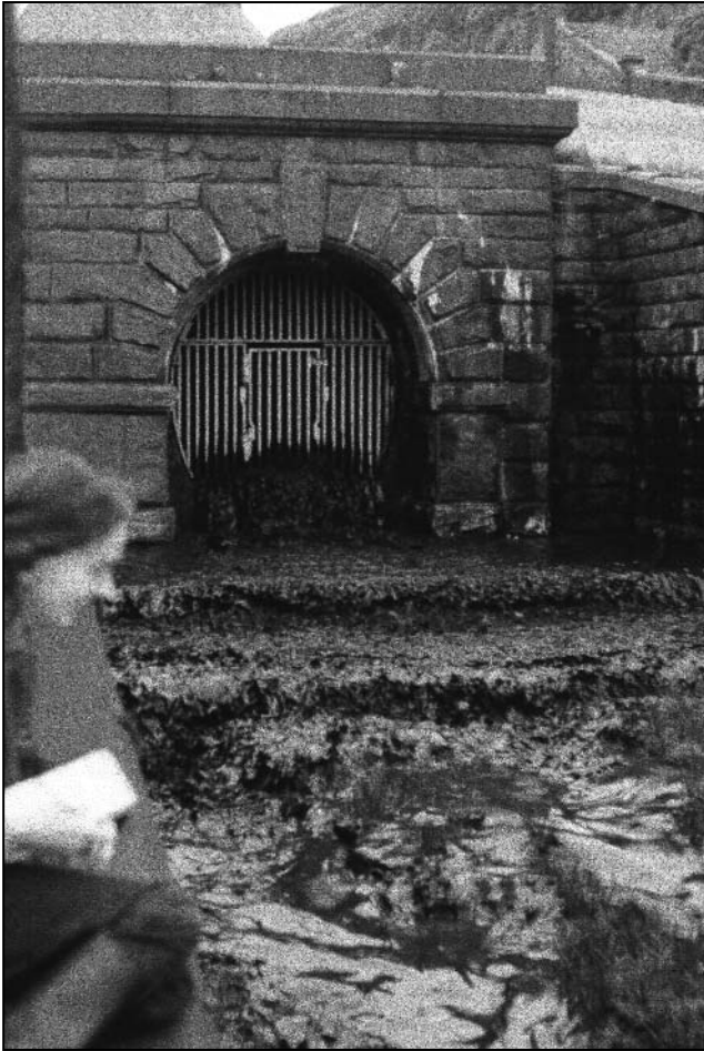
Figure 6. Sediment-rich water released on opening the bottom scour valve at Blakeley Reservoir, Yorkshire
