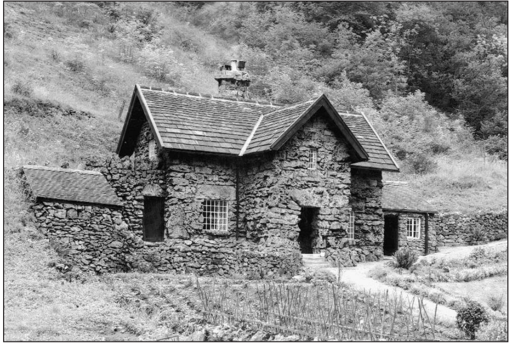
Figure 6. Marl Cottage, Via Gellia Valley, Derbyshire, constructed of large blocks of calcareous tufa quarried from the hills behind (BGS photo #A9125, 1957).
